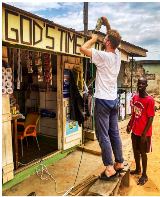
Julian installing with Valentine assisting
